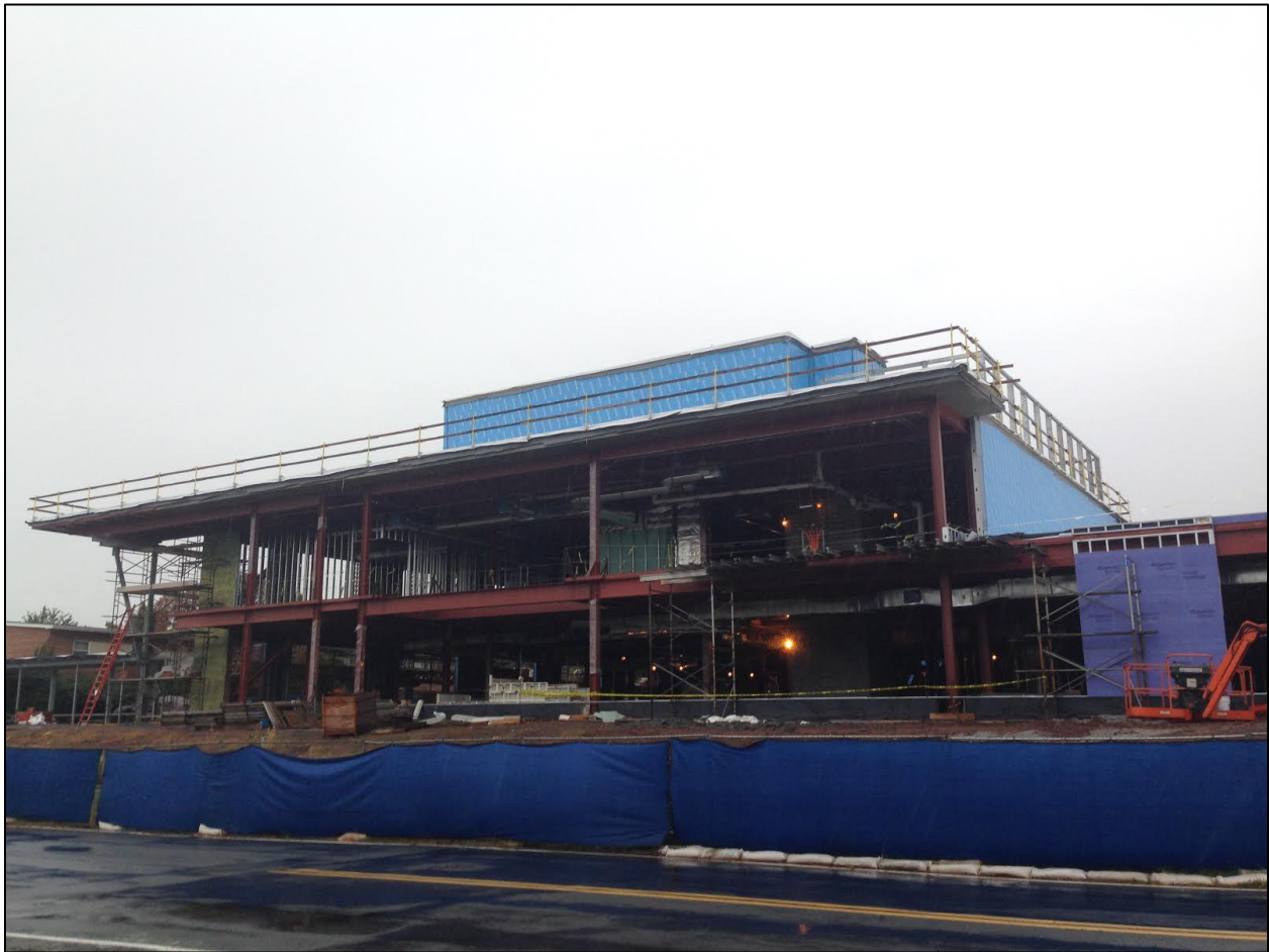
Figure 2 The 6 foot high fence around the construction site
